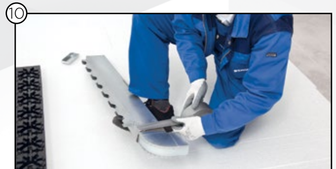
10 Sealing with floor duct tape (fabric lining)
