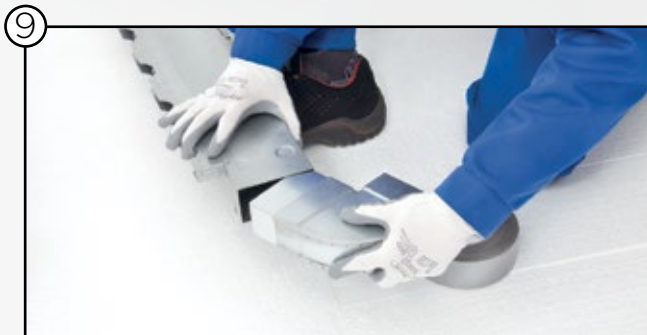
9 Installing shallow duct elbow
