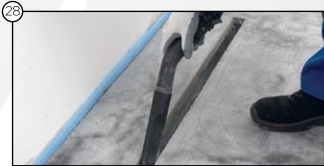
Cleaning the air outlet manifold
