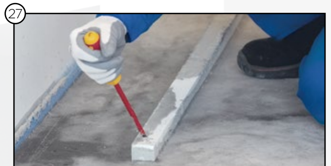
Removal of the air outlets screed protector
