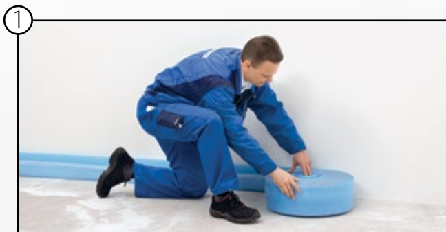
1 Install edge insulation strips
