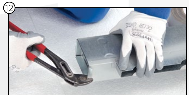
12 Secure lid by bending the holding lugs
