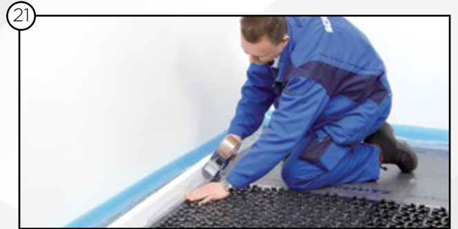
Taping the air outlet screed protector
