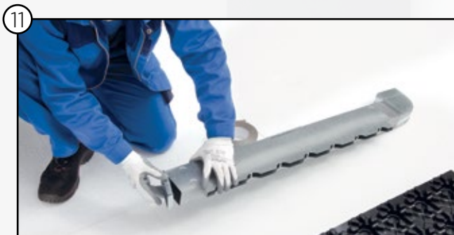
11 Closing the open side of the inlet manifold with lid
