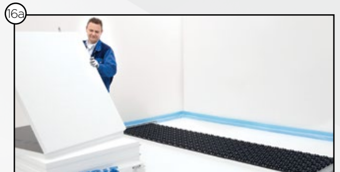
16a Laying the AIRCONOMY® folding panels
