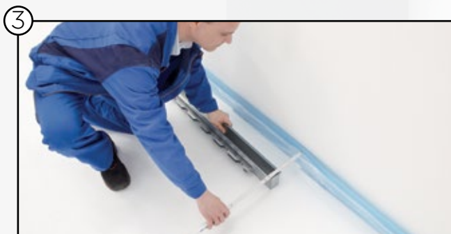
3 Position air outlet manifold
