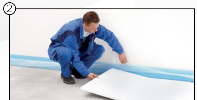
2 Lay sound insulation
