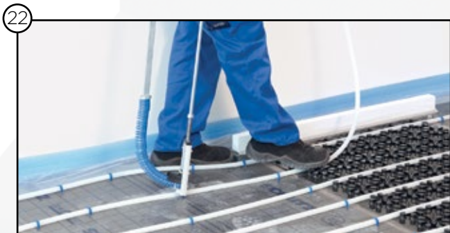
Securing the heating pipe
