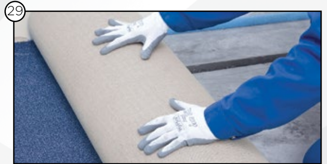
Laying of the floor covering
