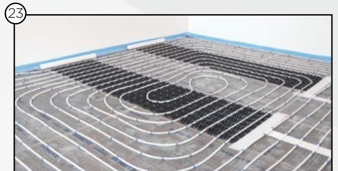
Heating pipe layout example
