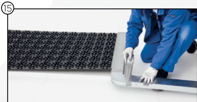
15 Mounting and taping the rest of the shallow ducting
