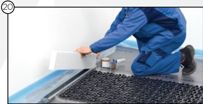
Fitting the air outlet screed protector
