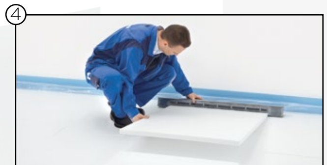
4 Lay distance panel to AIRCONOMY® system module
