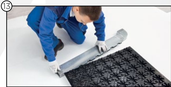
13 Mounting the inlet manifold onto the AIRCONOMY® system module
